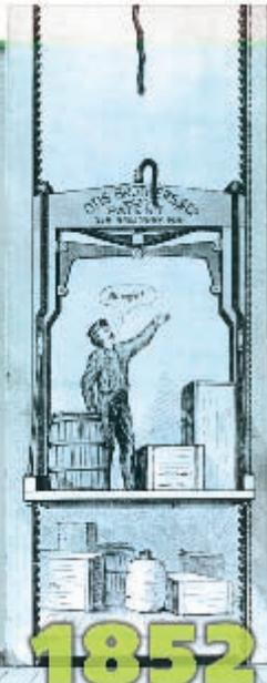
◀ **Safety Elevator** Elisha Otis develops a safety mechanism to prevent elevator cars from suddenly falling. He demonstrates his invention at an exposition in New York.
